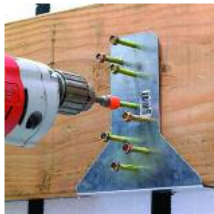
Fig. 3.18 – Installing a wood ledger with ICFVL.
