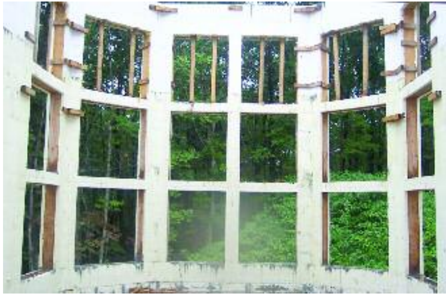
Fig. 3.3 – An ICF wall with several window openings during construction
