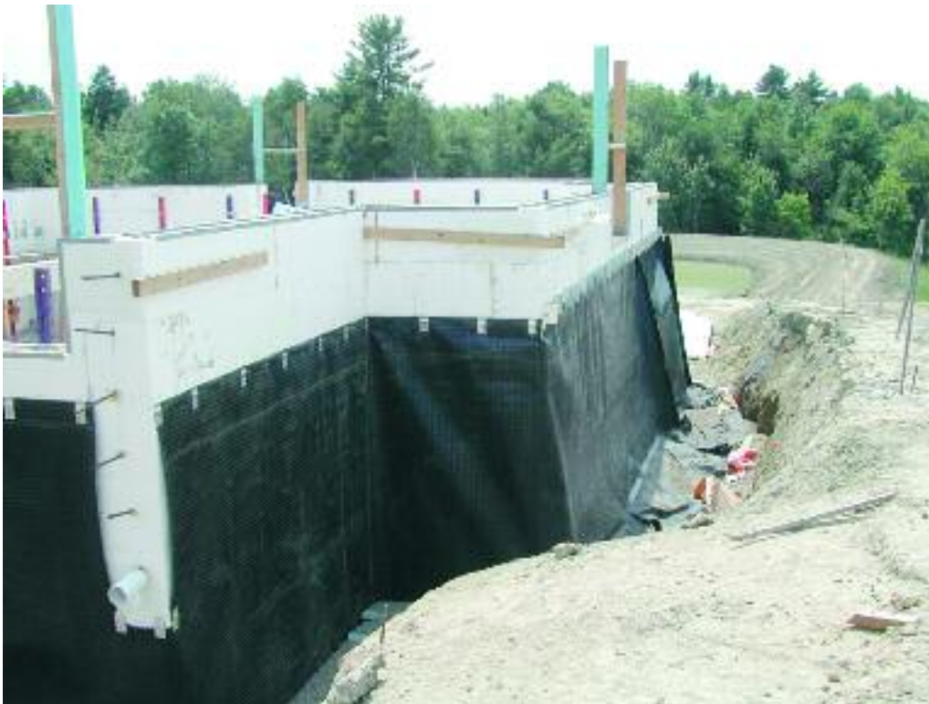
Figure 8.9 – Installed dimple sheet membrane
