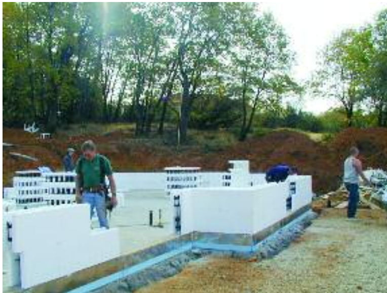
Figure 2.4 – Installing second course of ICF
