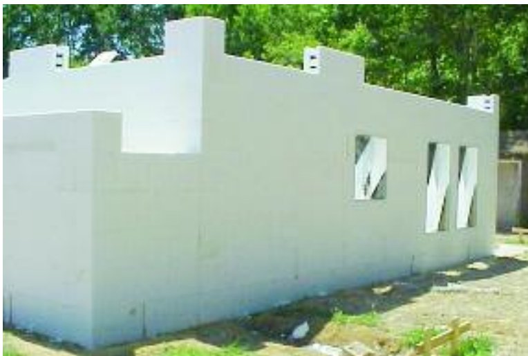
Figure 2.6 – Continuing installing block courses
