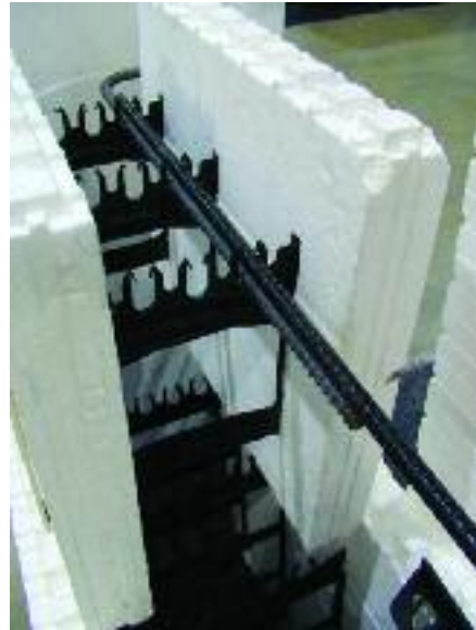
Figure 2.3 – Installing horizontal reinforcing steel and lap splicing
