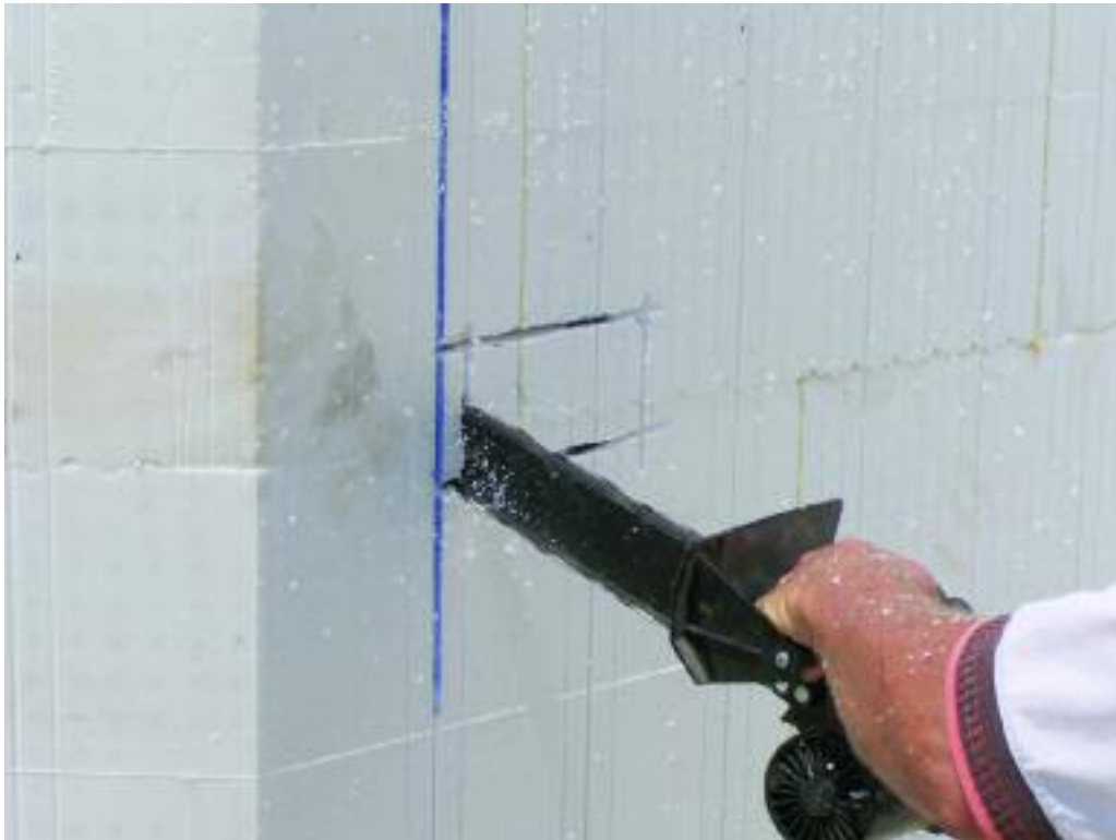
Figure 8.2 – Cutting a channel in the EPS panel using a chainsaw
