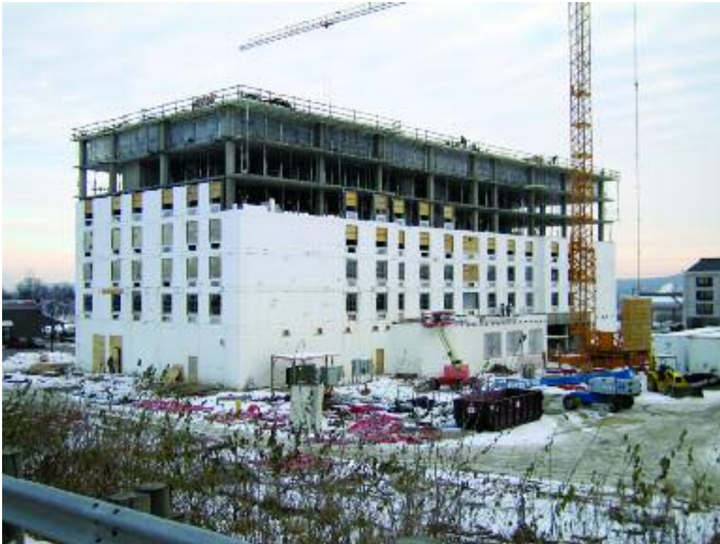
Fig. 3.2 – A multi-storey hotel being constructed with Amvic ICF
