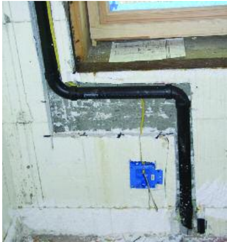
Figure 8.5 – Vent pipe embedded in the EPS foam
