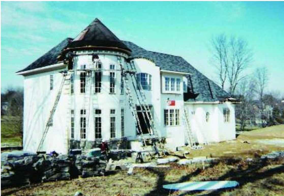
Fig. 3.1 – A custom home being constructed with Amvic ICF
