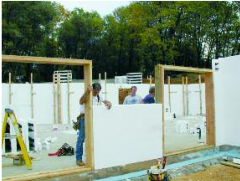
Figure 2.5 – Installing window and door bucks
