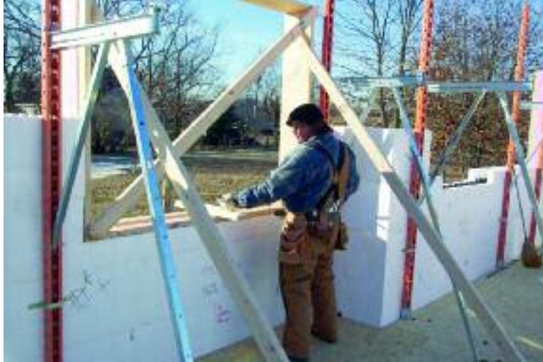
Figure 2.7 – Installing alignment and bracing system around the perimeter of the wall
