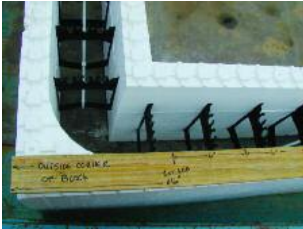
Figure 2.2 – Placing corner blocks first
