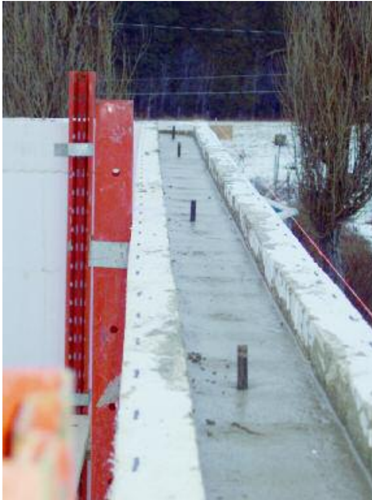
Figure 2.10 – Wet set anchor bolts in top course of upper floor
