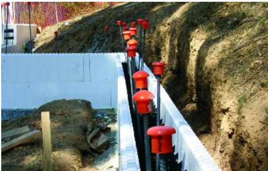
Figure 3.25 – Plastic mushroom caps on protruding steel bars
