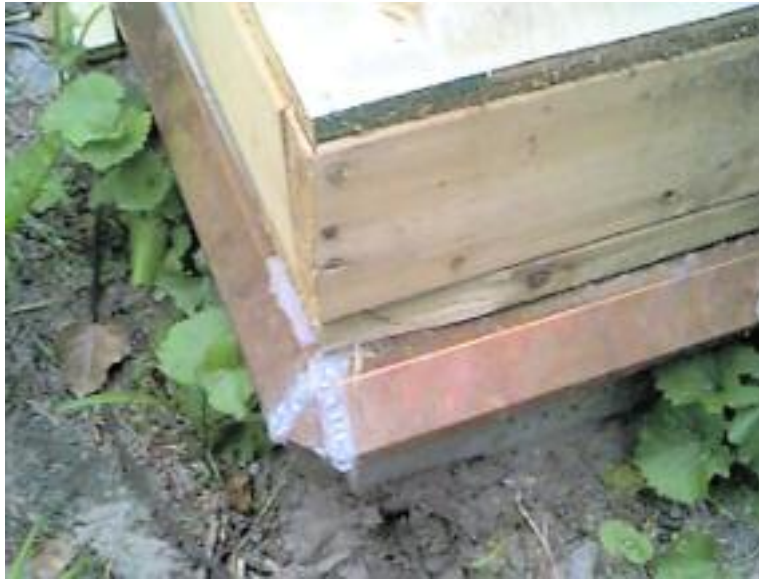
Figure 8.11 – Metal termite shield using copper metal on top of foundation wall. Copyright ©1998-2005, Urban Entomology Program, University of Toronto www.utoronto.ca/forest/termite/termite.htm
