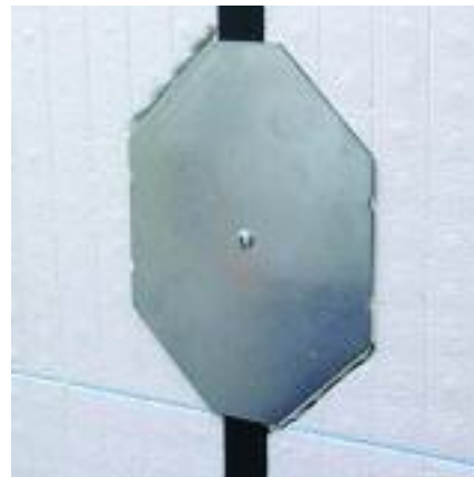
Fig. 3.17 – ICFVL installed on ICF wall.
