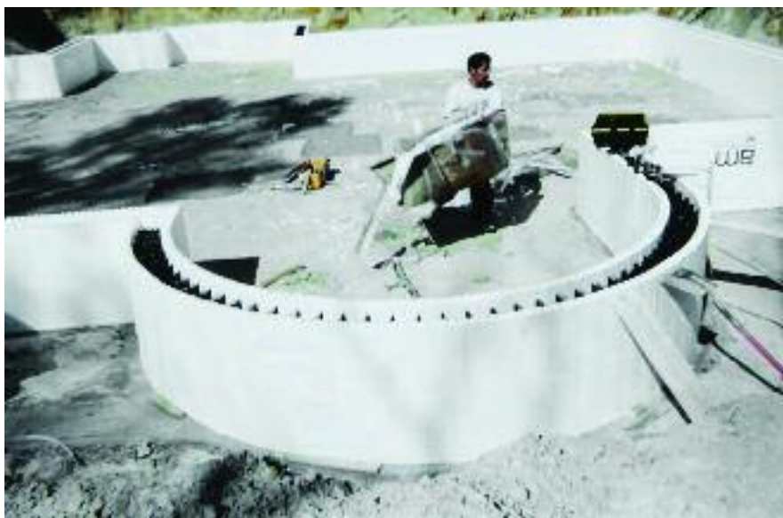
Fig. 3.4 – A curved ICF wall during construction
