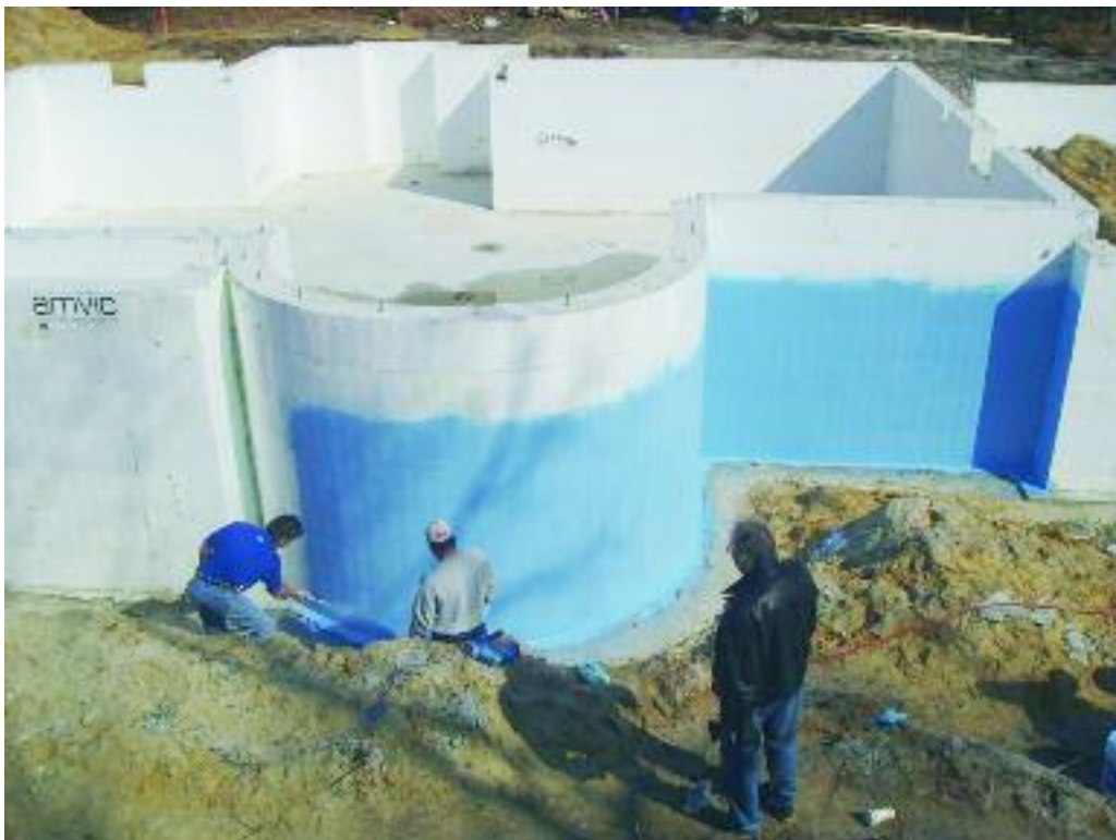
Figure 8.7 – Spraying liquid applied membrane on Amvic ICF
