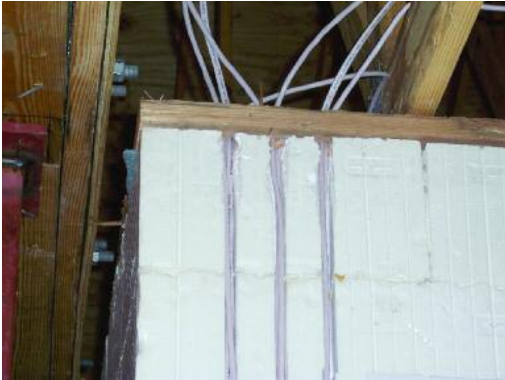
Figure 8.3 – Embedding Romex into the EPS panels
