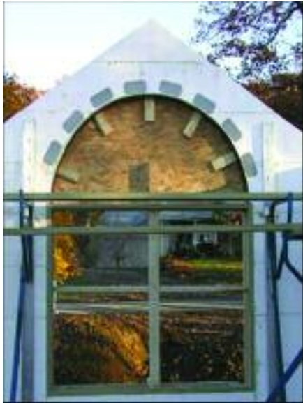
Fig. 3.11 – Grapplers installed in an ICF wall.
