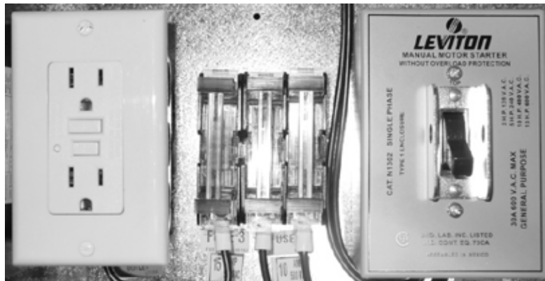
Figure M2 - Factory Wired Convenience Outlet
