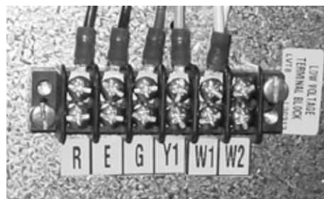
Figure T1 - Example Low Voltage Terminal Block
