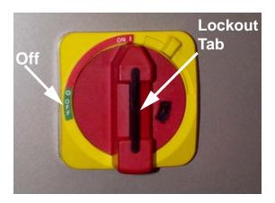
Figure 1-1 Rotary Disconnect Switch
